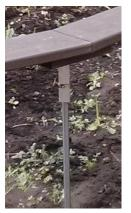
A stainless steel hose clip holds the bracket and allows vertical adjustment to compensate for ground movement.
